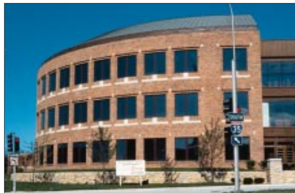
A water-based water repellent used on a church complex in Kentucky had to be chemically removed and replaced with a new material because excess surfactant in the original material left a blush appearance on the surface. Designed to meet limits on volatile organic compounds (VOCs), properly formulated and applied water-based products will not discolor.
