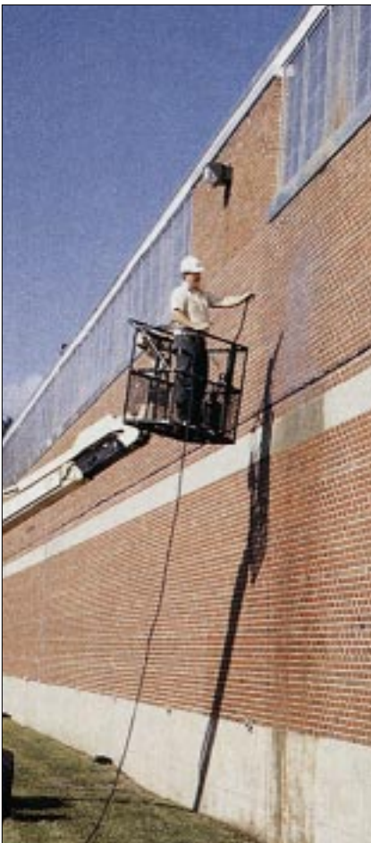
The Brick Institute of America now states that water-repellent coatings may be appropriate for use on brick masonry in certain situations.
